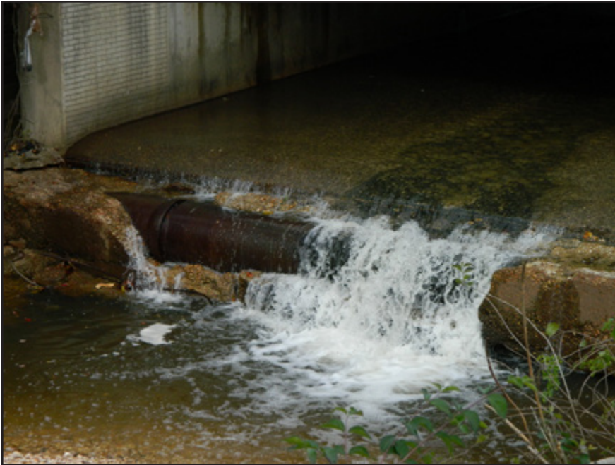
Exposed pipe and bank undercutting on Winkle Doodle Branch at the MD 210 Bridge
